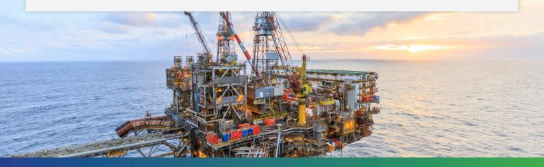
Apache's adoption of AIM™ inspection service on the Beryl Alpha platform has significantly reduced offshore inspection hours of the topside structure whilst enhancing the quality and availability of inspection data. The overall offshore inspection times were slashed from six months to just six weeks, whilst the inspections costs were reduced by more than 20 per cent.
