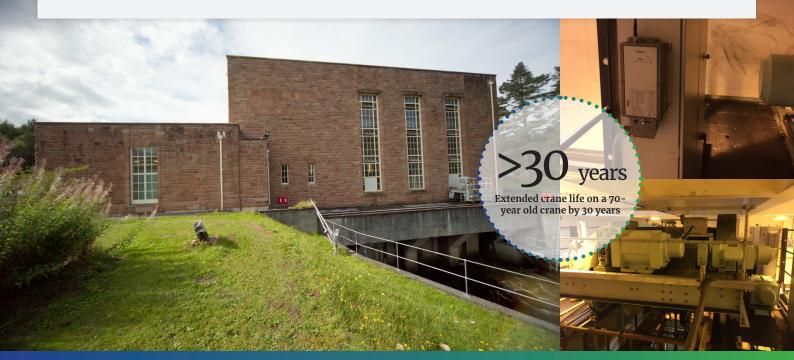
The Grudie Bridge Power Station is located at Loch Luichart in the Scottish Highlands. The overhead crane currently in operation dates back to 1946 and was last subject to a maintenance overhaul and electrical upgrade in 1994. Client: Scottish and Southern Energy (SSE)
